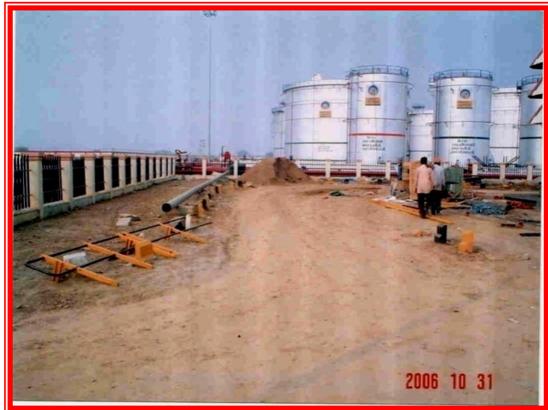
COMPLETION OF STORAGE TANK AT PYALA (HARYANA)
