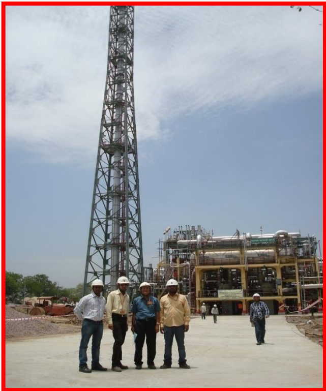
COMPLETION VIEW OF SRU-IV AT MATHURA REFINERY
