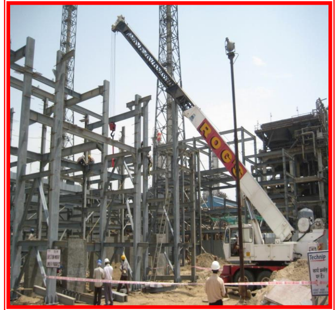
STEEL STRUCTURE ERECTION AT SRU-IV MATHURA REFINENRY
