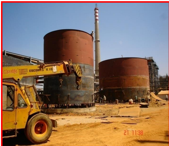
FABRICATION OF STORAGE TANK AT PYALA (HARYANA)
