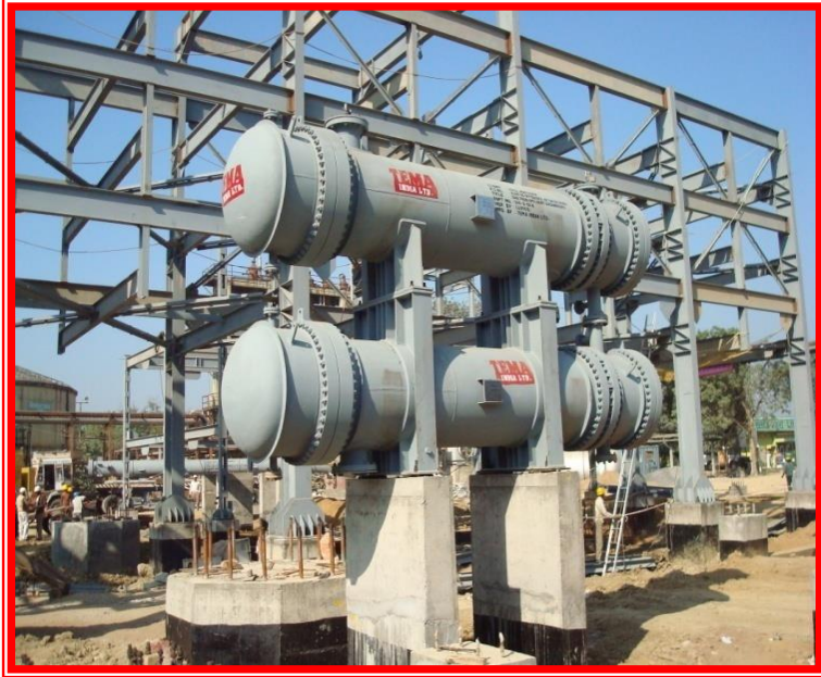
EQUIPMENTS ERRECTION AT MSQ EURO-IV,MATHURA REFINERY
