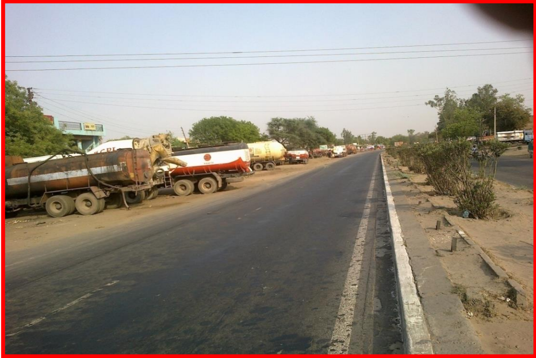
ROAD WORK AT IRCON CAMP CHAUMAH, DELHI MATHURA HIGHWAY
