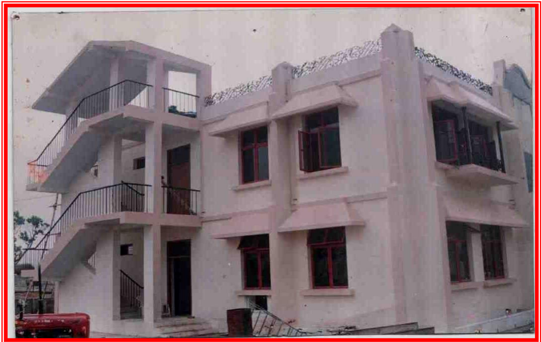
MMMPL EXTENSION PROJECT AT B.P.C.L. CONTROL ROOM MATHURA
