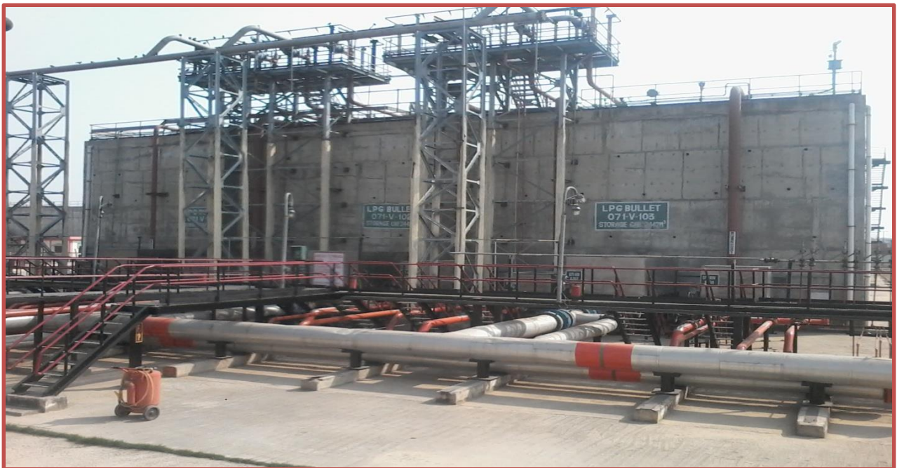
G.R. ENGINEERING 6 NOS. MOUNDED BULLETS JOB AT MATHURA REFINERY.
