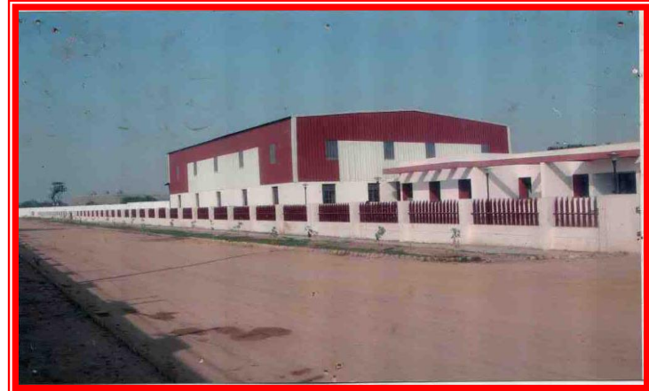
CONSTRUCTION OF WARE HOUSE B. P. C. L. AT LONI
