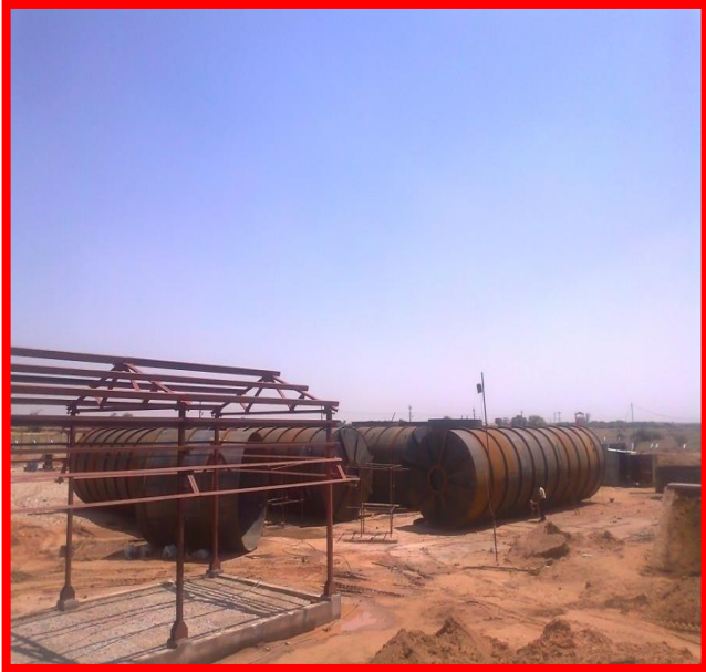
FABRICATION OF ATF STORAGE TANKS AT PHALAUDI BPCL SITE
