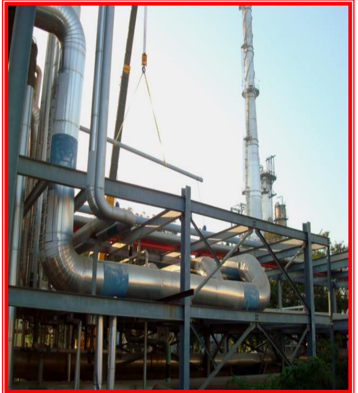
O.S.B.L. PIPING ERECTION IN MATHURA REFINERY
