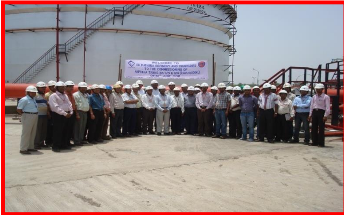
COMPLETION OF CIVIL WORK TANK NO 124 AT MATHURA REFINERY
